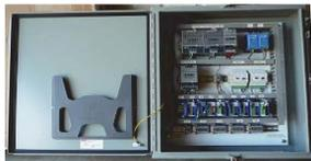
*Stack Unit:* This unit provides redundant 24VDC power to the emission probes and contains ioPro IO units to redundantly read the 4 to 20mA outputs from the probes. Also, redundant DI units monitor various status points. Up to 20 channels can be supported
