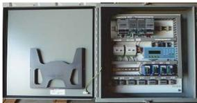
*Control Unit:* This unit is connected to the Stack Unit via redundant fiber optic cables. It contains a redundant power supply to an IOS Controller with custom software to read the redundant IO, process the data, and output the results as 4 to 20 mA outputs to the emission analyzer. Error logging and reporting is done via an intuitive user interface on enclosed LCD display. An error output is provided that feeds into the overall plant monitoring system for trouble notification.
